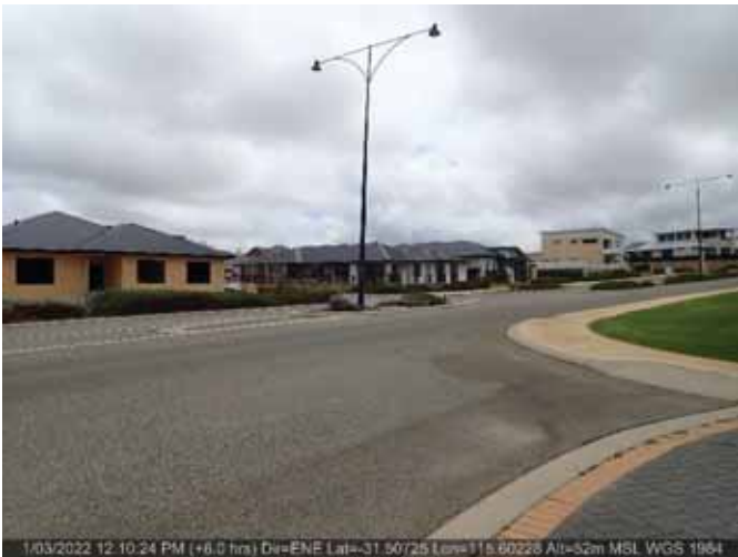
Photo ID: Photo 5 The established suburb adjacent to the development site.
