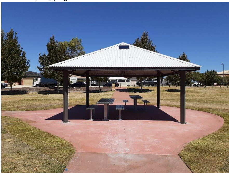
Eiffel Park, Tapping – Shelter Renewal
