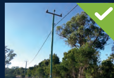
Compliant: cleared buffer zone around power poles
