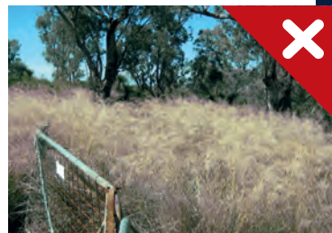
Non-compliant: no fire break installed inside boundary fence
