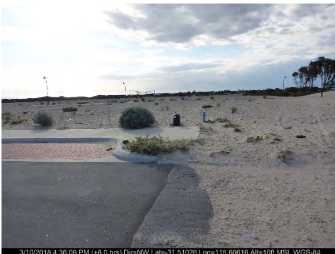
3/10/2018 4:36:09 PM (+8.0 hrs) Dir=NW Lat=-31.51026 Lon=115.60616 Alt=10ft MSL WGS-84 Photo ID: Photo 9 The cleared land and associated road infrastructure south-east of the development site.
