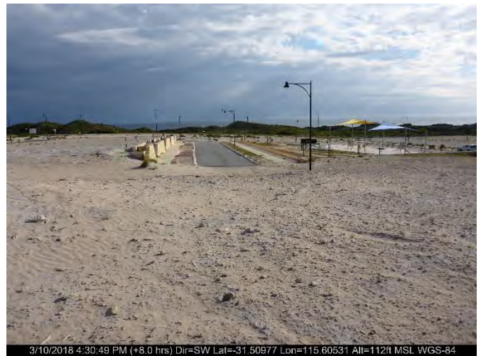
3/10/2018 4:30:49 PM (+8.0 hrs) Dir=SW Lat=-31.50977 Lon=115.60531 Alt=112ft MSL WGS-84 Photo ID: Photo 8 The cleared land and associated road infrastructure east of the development site.
