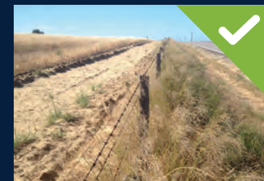
Compliant: mineral earth fire break
