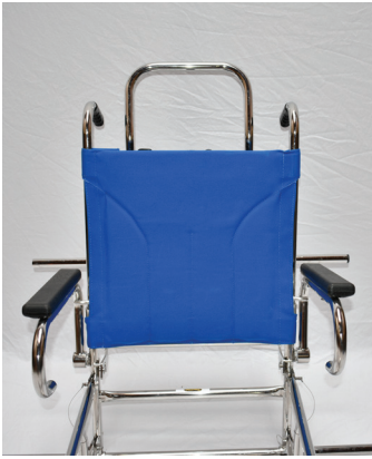
Install seat back pad and attach buckles.
