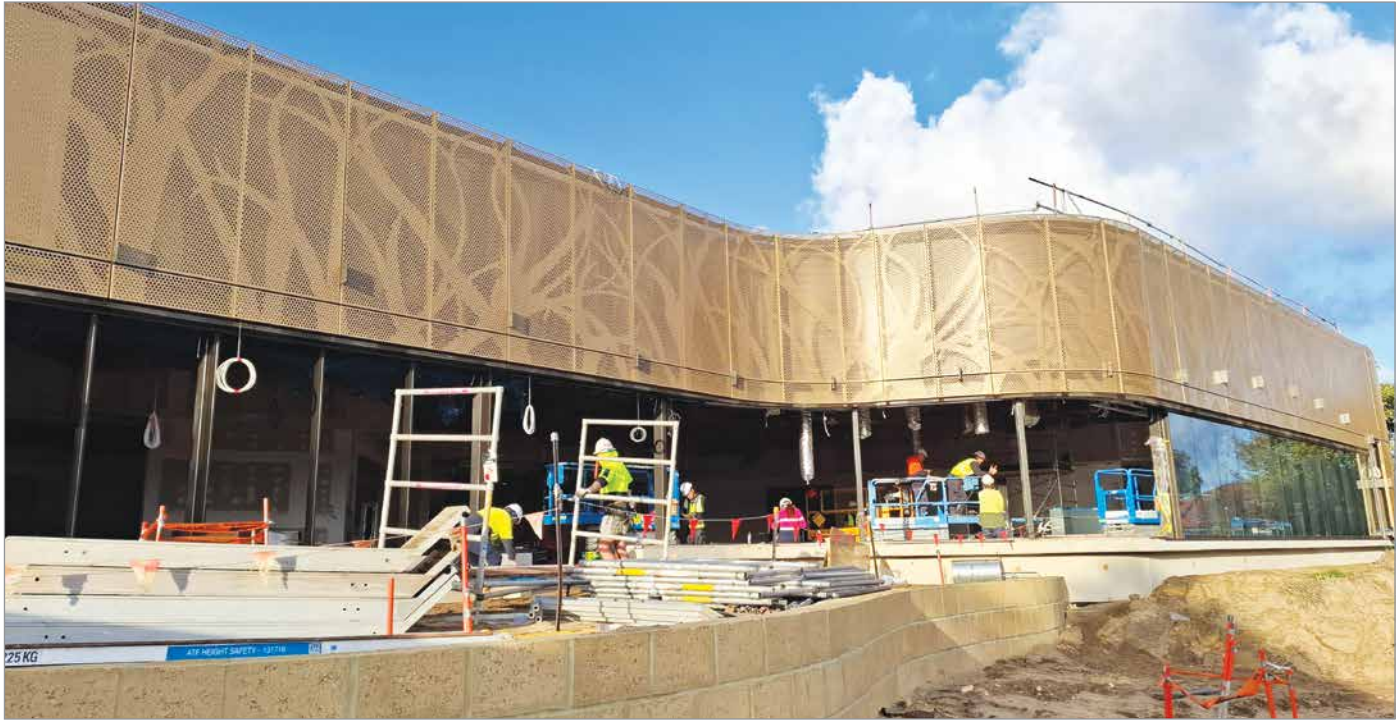
Dordaak Kepup's eye-catching perforated cladding was installed in June.
