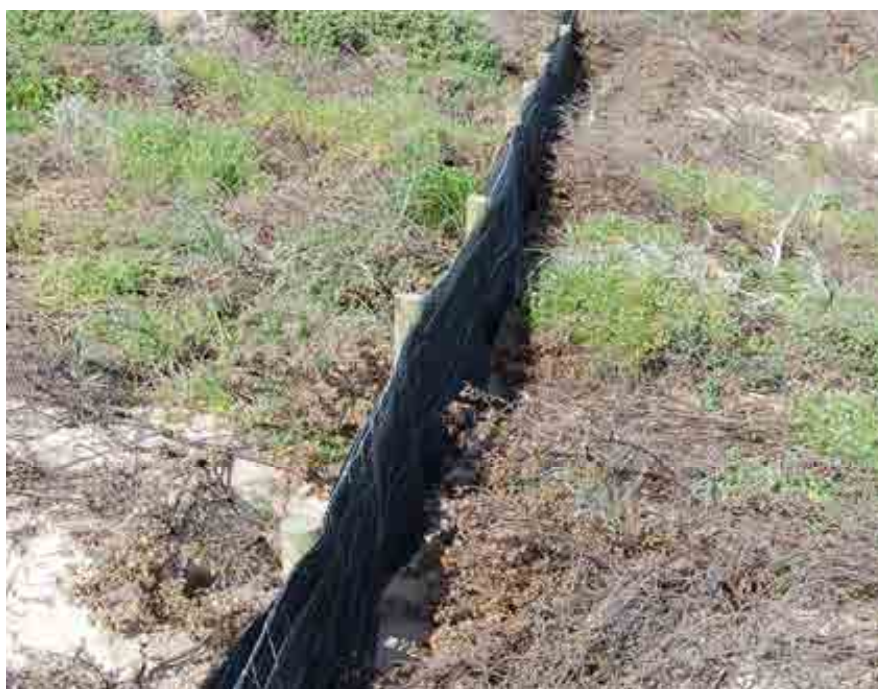
Plate 2: Example of Sand trap fencing used in a coastal dune environment
